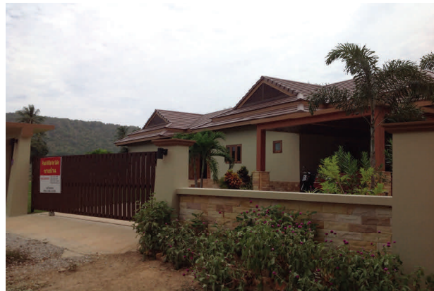
Constructed with 15cm wide Super Blocks offering high insulation from heat. Roof insulated and tiled with CPAC flat tiles.
